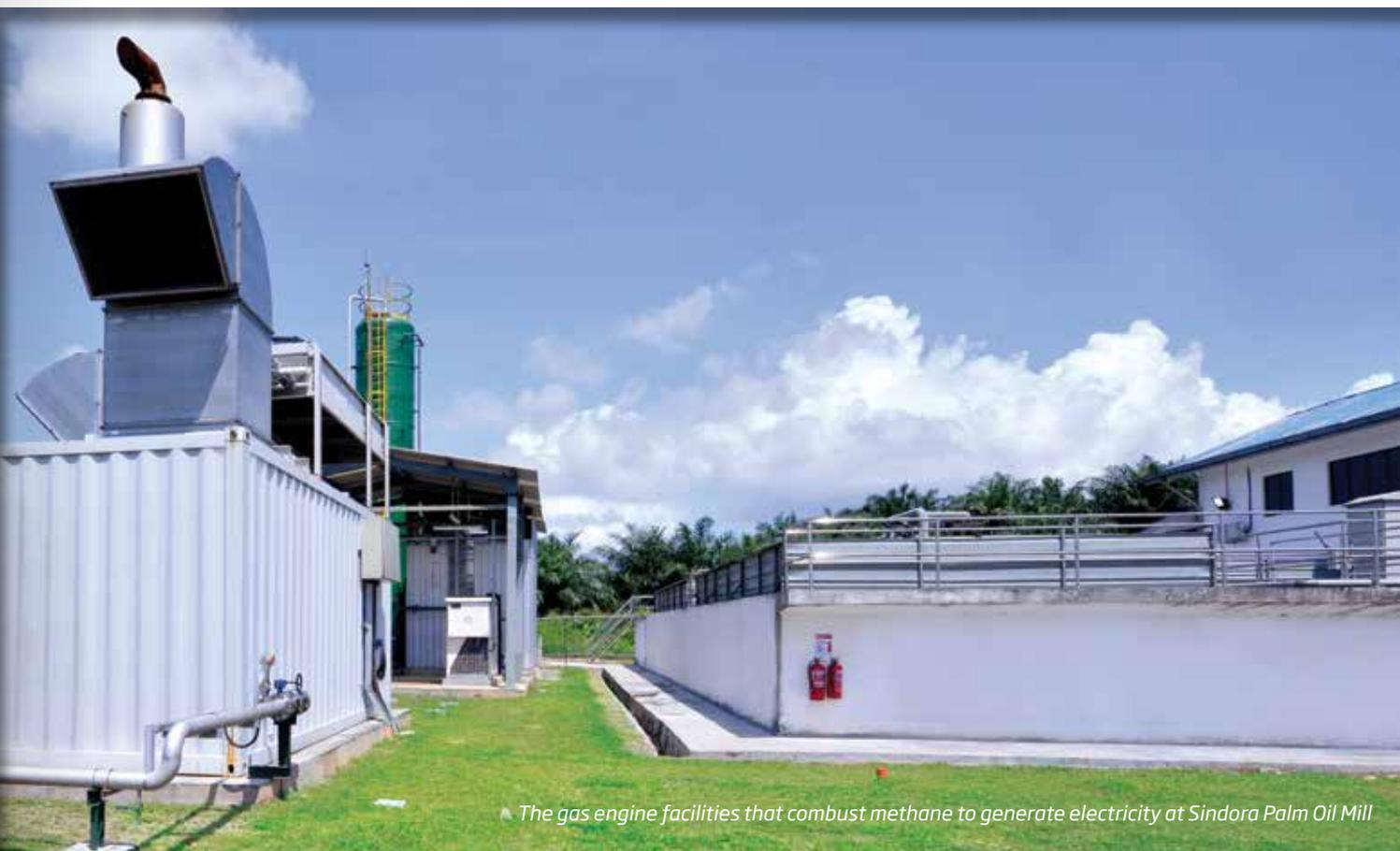
The gas engine facilities that combust methane to generate electricity at Sindora Palm Oil Mill
